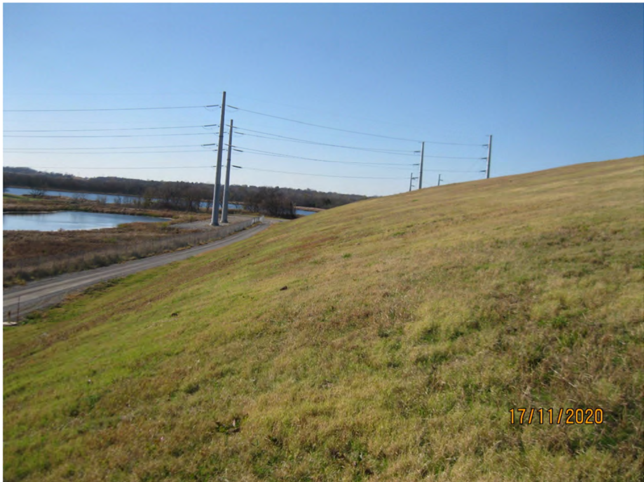
Figure 4-2 Final Cover on CCR Material – South Slope - Looking West
