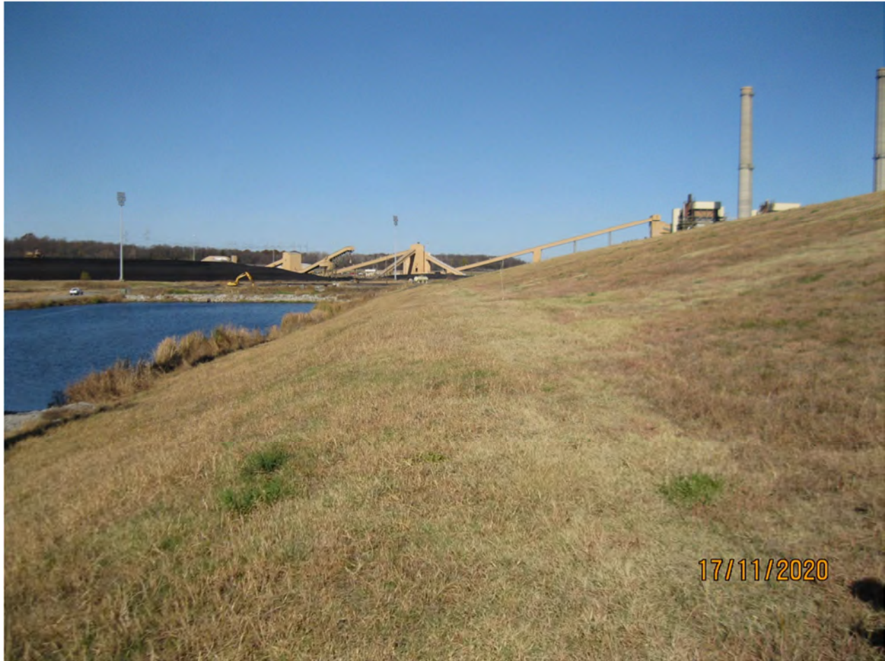
Figure 4-1 Field Photo of West Embankment, Looking North
