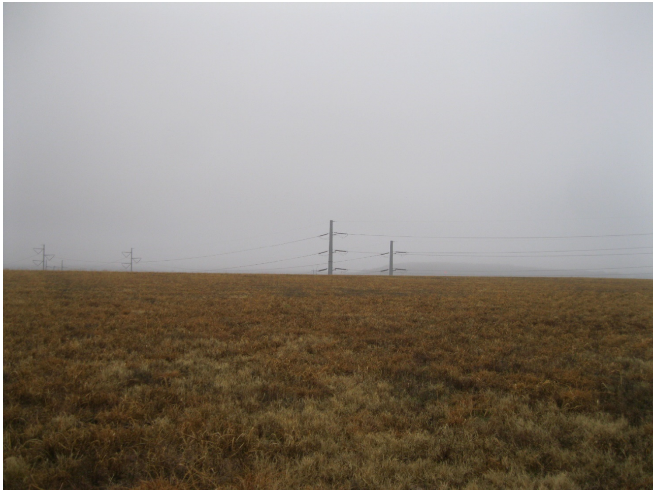
Figure 4-3 Final Cover on top of CCR Material – Top of Landfill from Center looking Southwest
