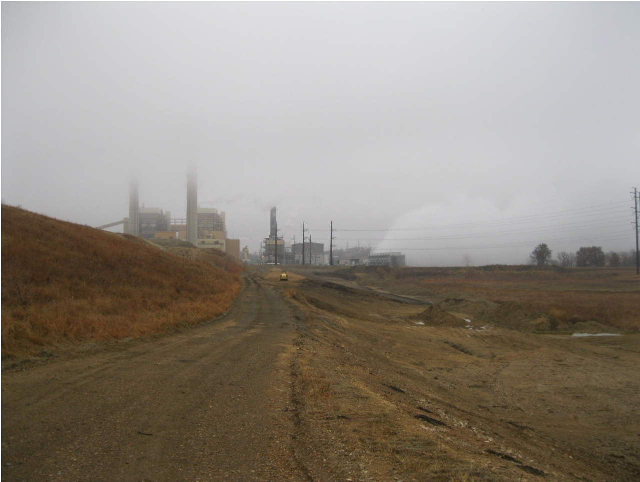
Figure 4-3 East CCR material with new embankment construction, South Looking North
