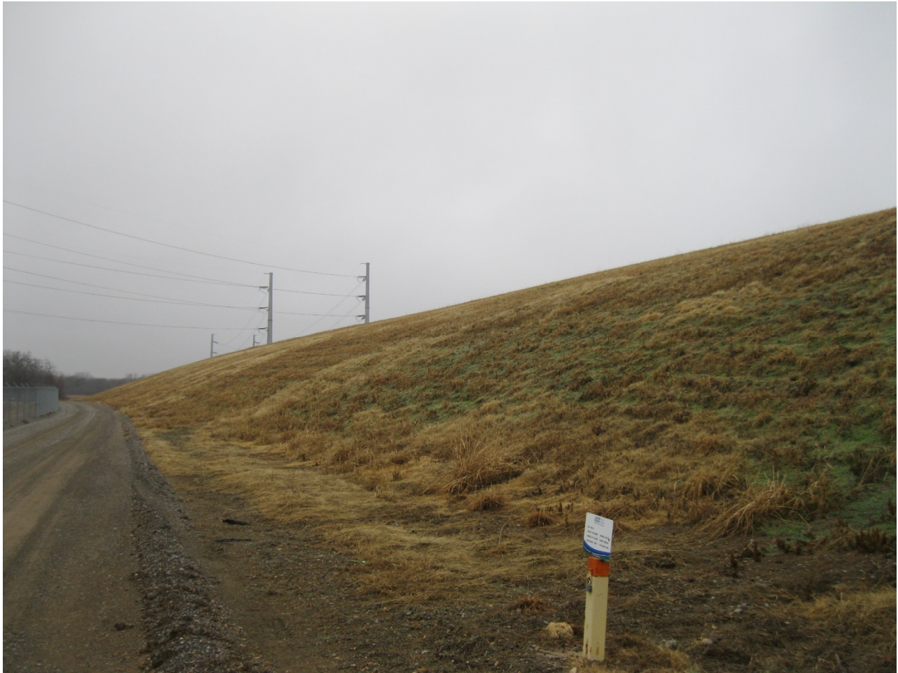
Figure 4-2 – South CCR Slope and Embankment with Vegetation Cover. East Looking West.
