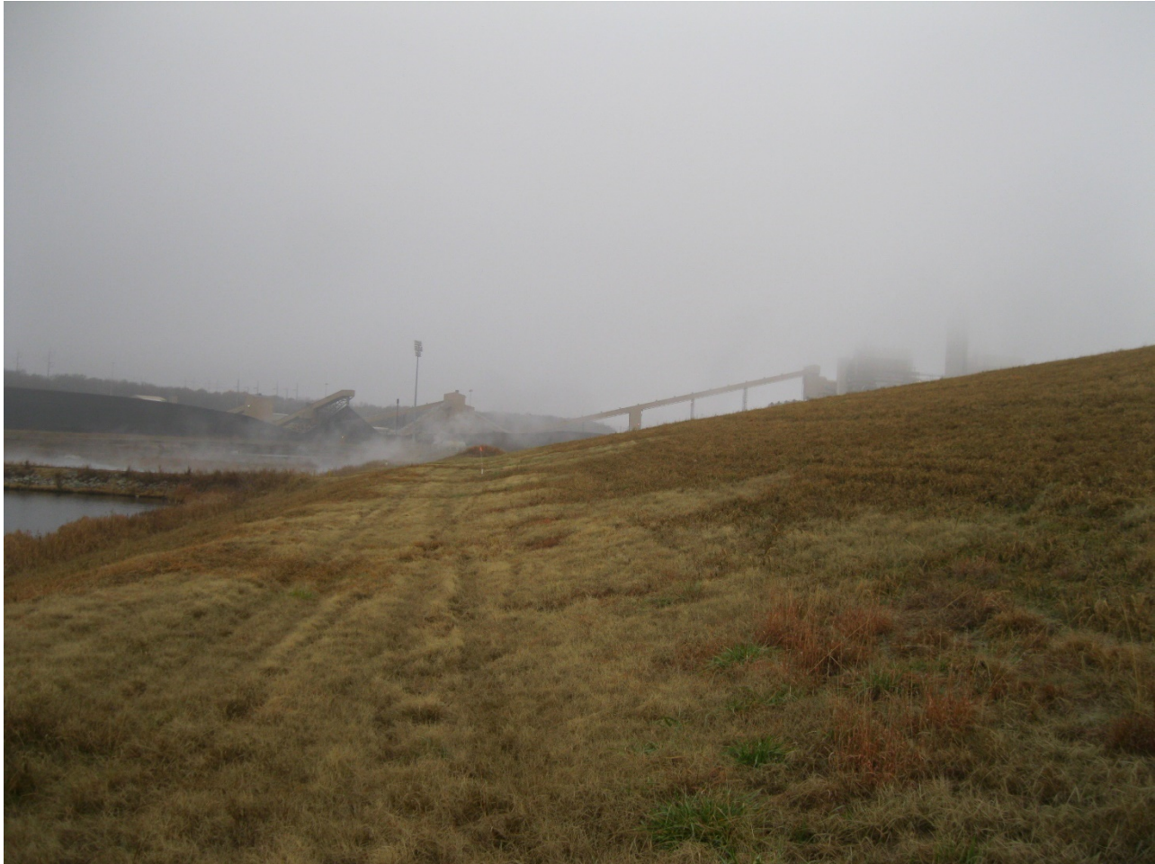
Figure 4-1 – Crest of West Embankment, Center Looking North.
