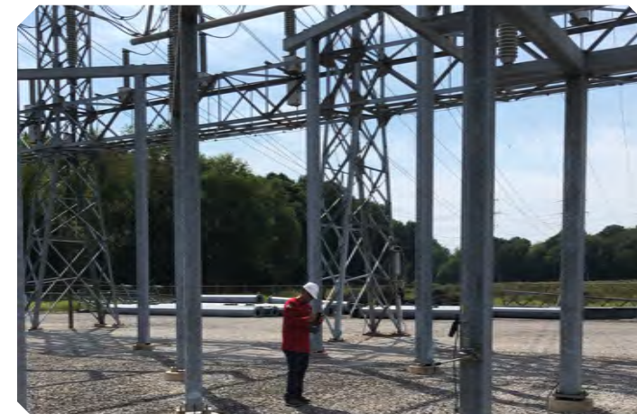
Performing a substation inspection
