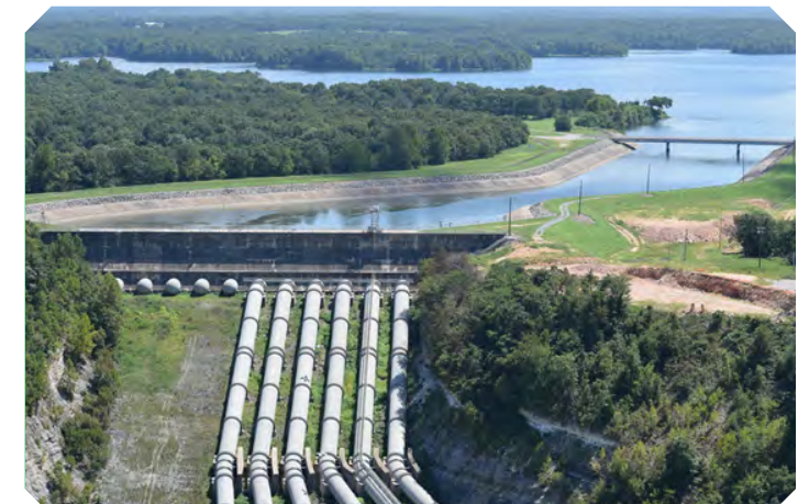
W.R. Holway and GRDA’s Salina Pumped Storage Project
