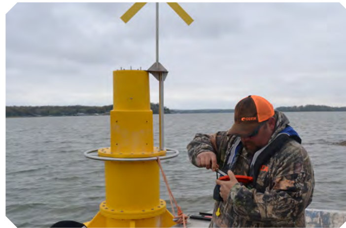
Shane Johnston works to install a navigation buoy
