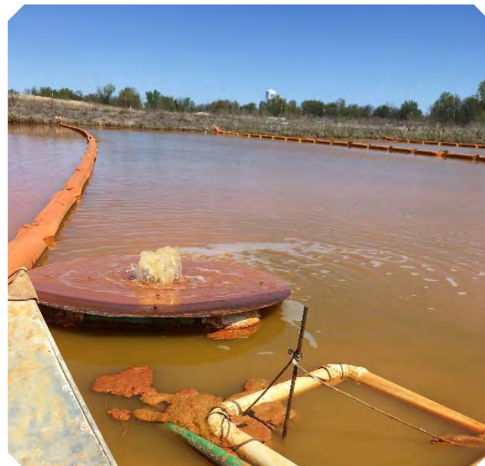
A float-mix aerator in a passive treatment pond
