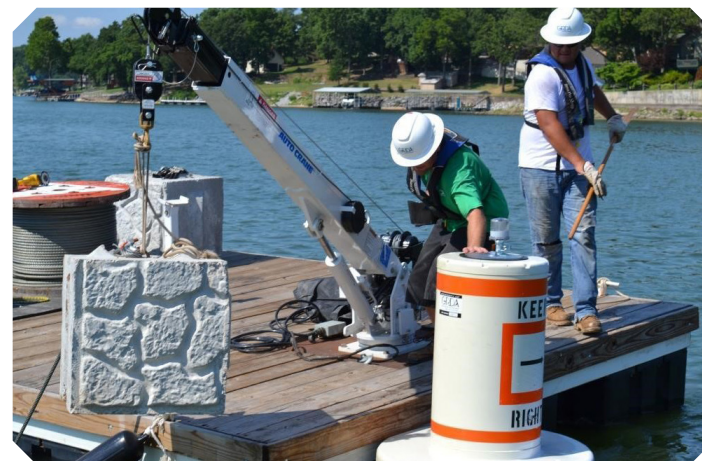
The shoreline management crew installs a buoy
