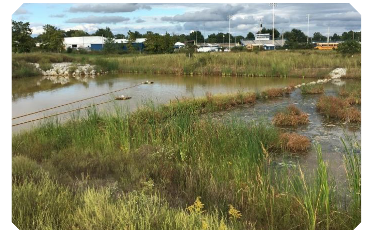
Southeast Commerce passive treatment system (PTS)
