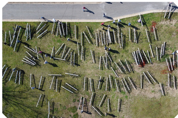
An aerial photo of the structures built in 2022
