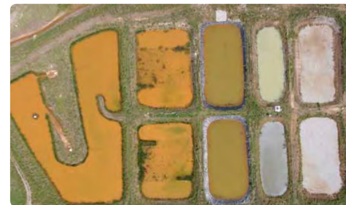
Aerial view of Meyer Ranch Passive Treatment System
