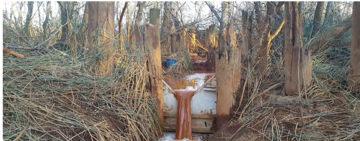
A weir installed in January 2019 to measure flow of mine drainage sources contributing to a nearby wetland
