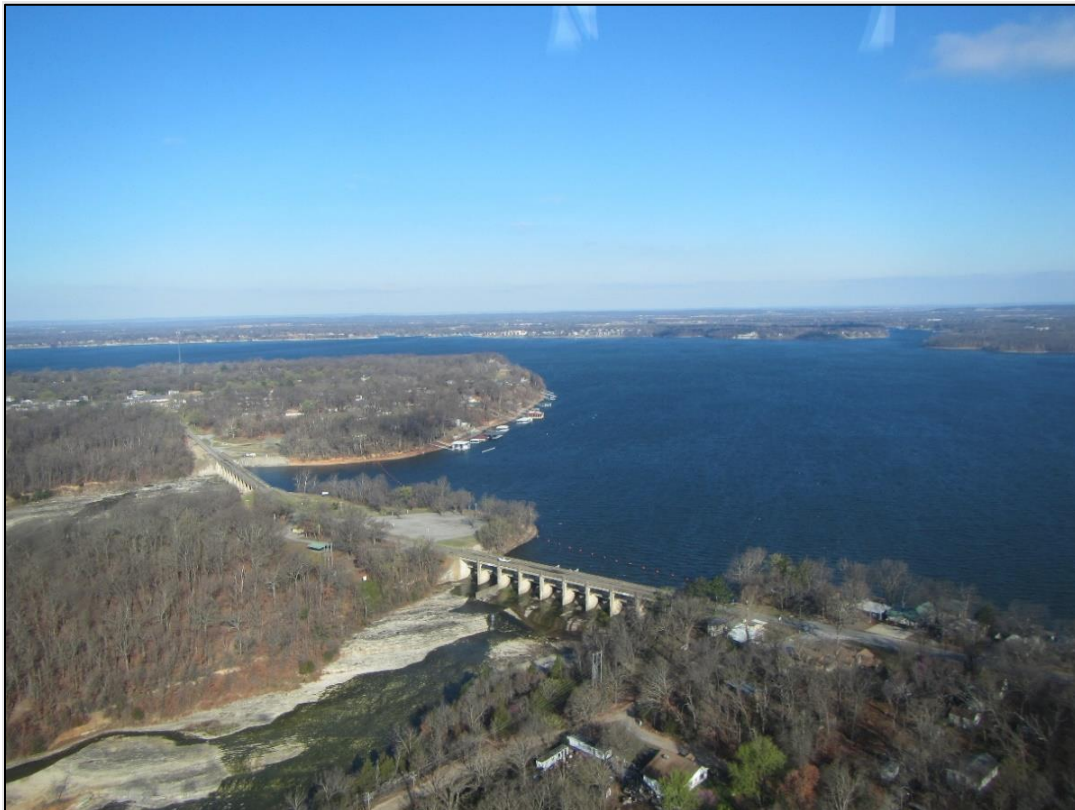
Figure 3.10.1-3 Pensacola Dam East Spillways and Grand Lake Looking Northwest
