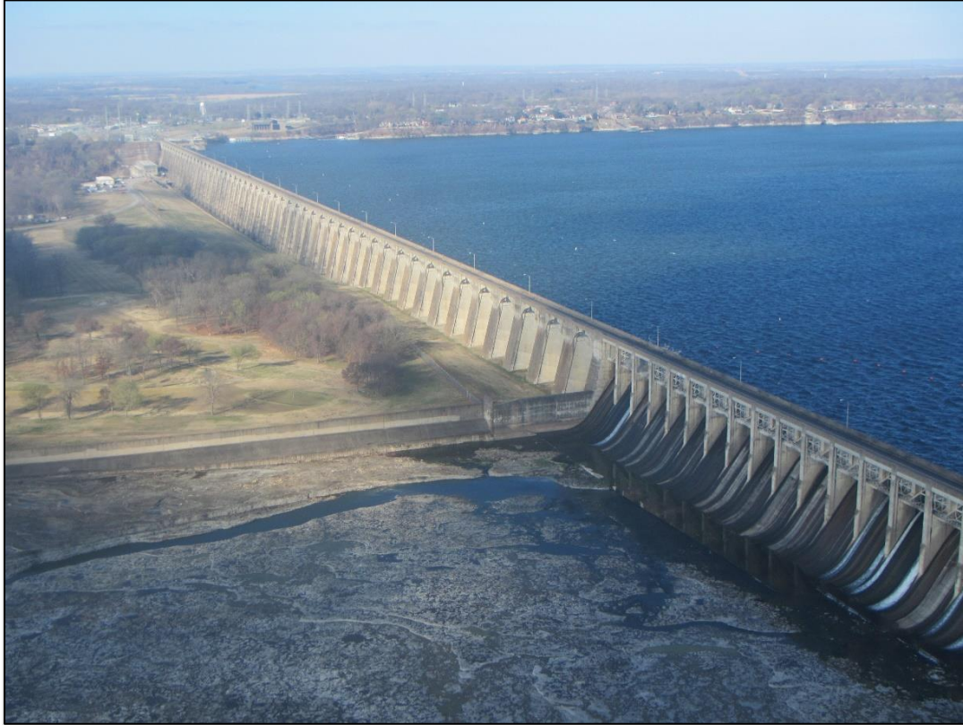
Figure 3.10.1-2 Pensacola Dam Looking West
