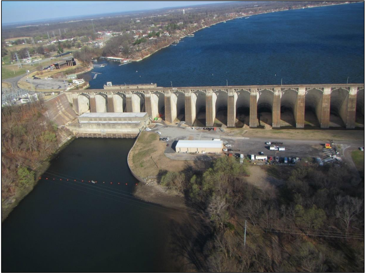
Figure 3.10.1-1 Pensacola Dam, Powerhouse and Tailrace Looking Upstream
