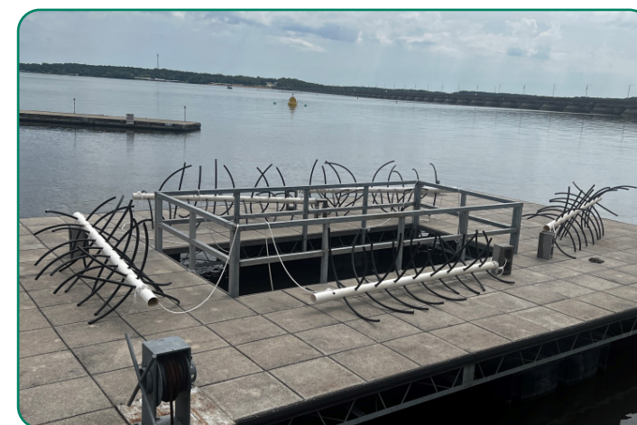
New habitat being installed at a GRDA courtesy dock
