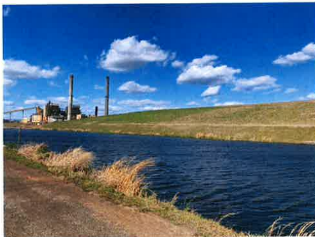
Figure 4.10 View of Vegetative Cover on West Sloped Side of Ash Landfill
