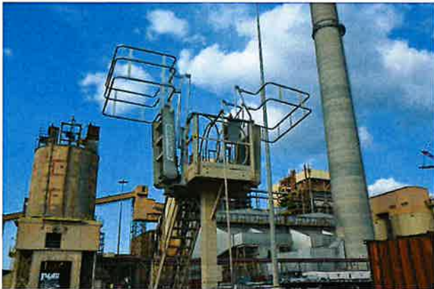
Figure 4.6 Truck Wash Station for Fugitive Dust Control
