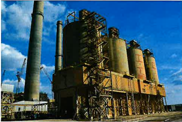
Figure 4.1 Ash Storage Silos with Partially Enclosed Truck Loading Bay
