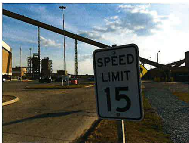
Figure 4.11 Example of posted 15 mph speed limit, with ash storage silos in background
