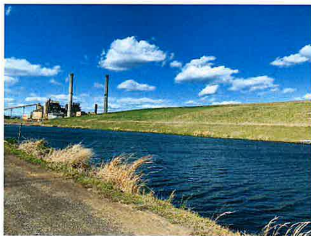
Figure 4.10 View of Vegetative Cover on West Sloped Side of Ash Landfill
